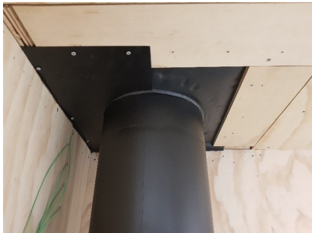
Photo 3: SabetoFLEX water vapour membrane below penetration, during installation
